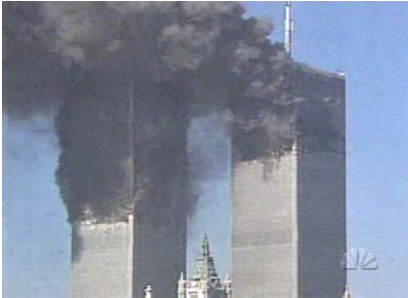
Figure 21.1.: Collapse Initiation: NBC video, frame 61
