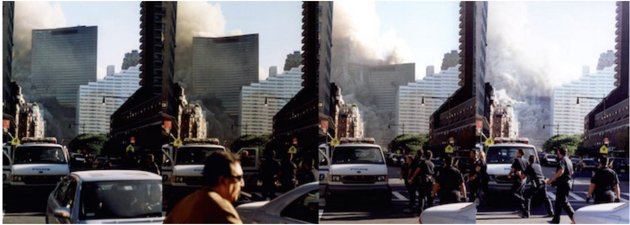
Figure 1.5 The collapse of WTC 7 at 5:20 PM (source unknown).
